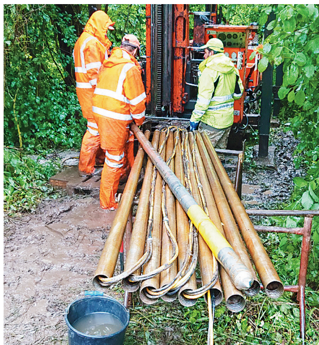
Fig. 2 Equipment necessary for the performing of dilatometer tests in boreholes.
