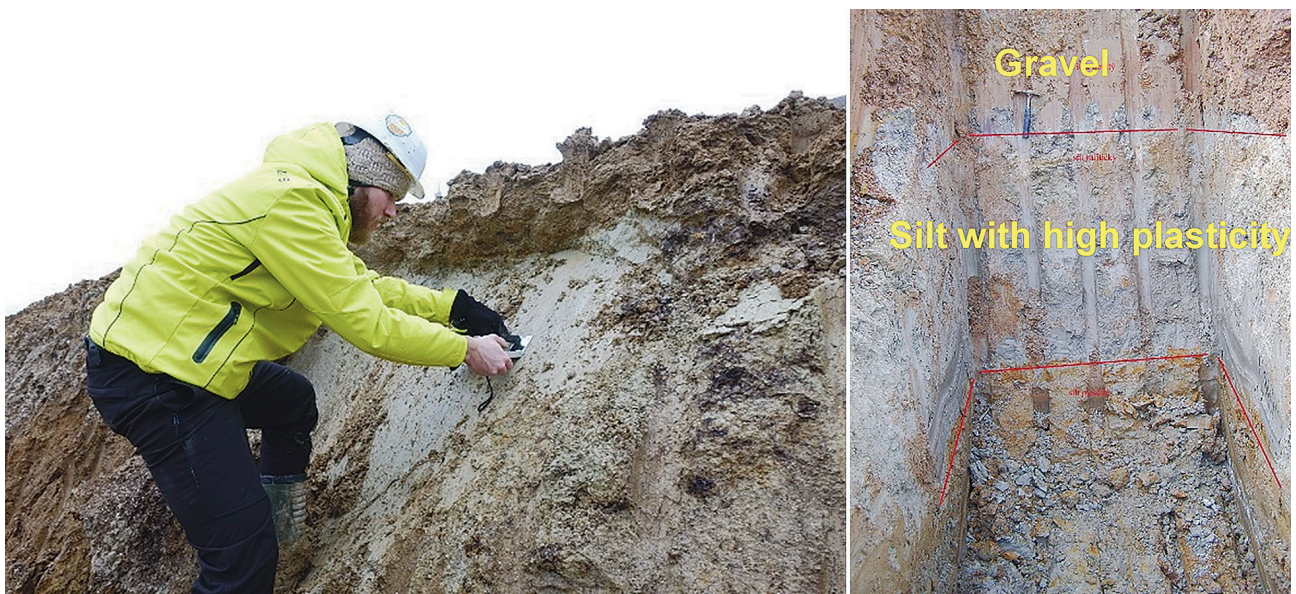
Fig. 6. Slip surfaces in the excavation of the cuts and the excavated shaft.
