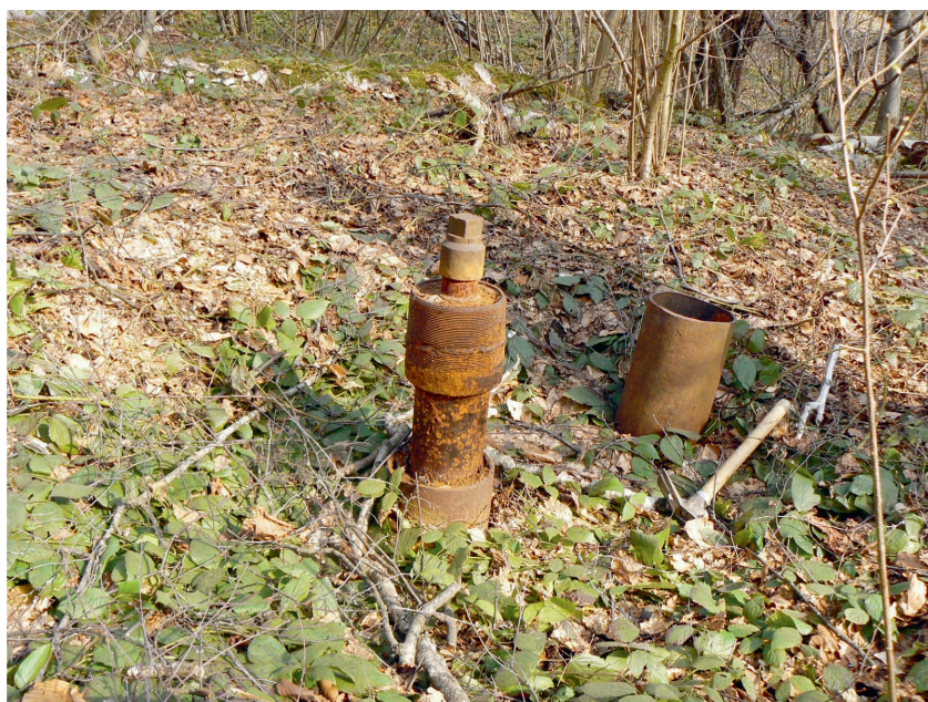
Fig. 3. Armature remnants from an old well of the Miková well series drilled in 1911–1943. (Photo by the first author; July 2010).
