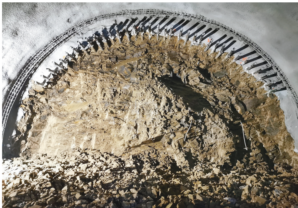
Fig. 4: Sandstones at the headwall of the Bikoš tunnel
