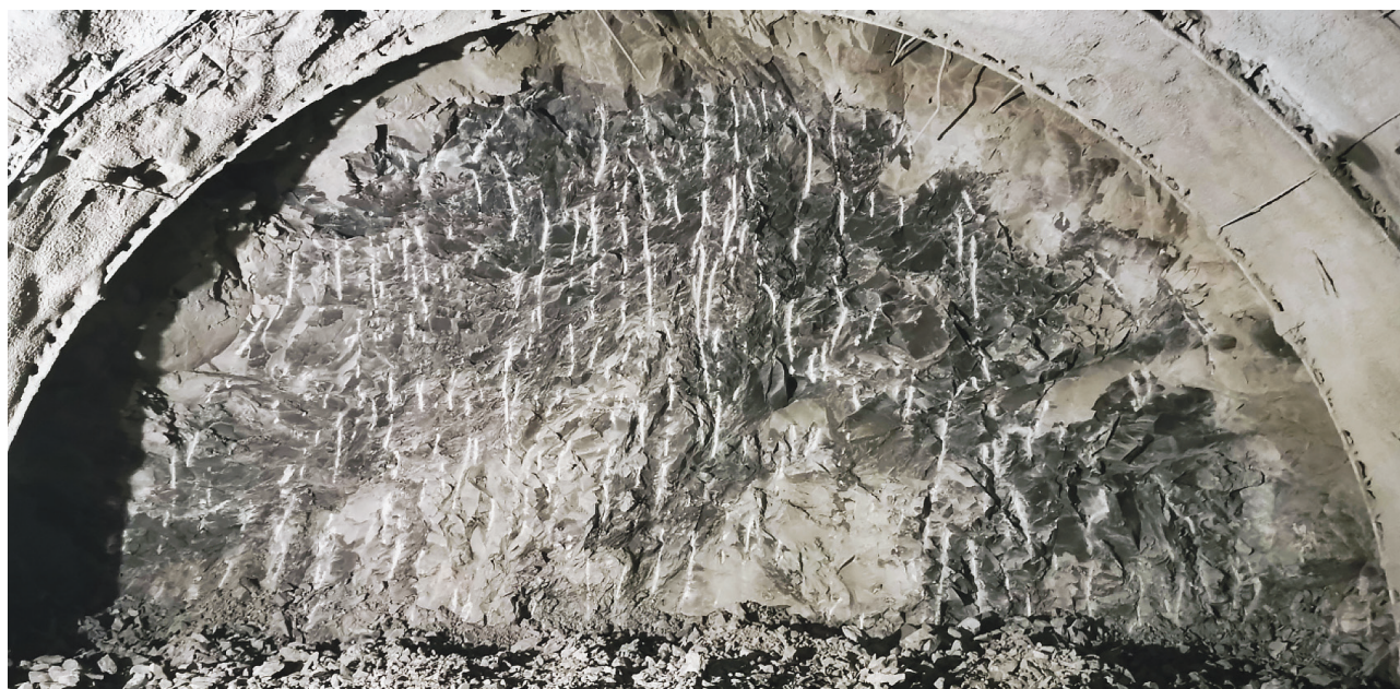
Fig. 3: Claystones at the headwall of the Okruhliak tunnel
