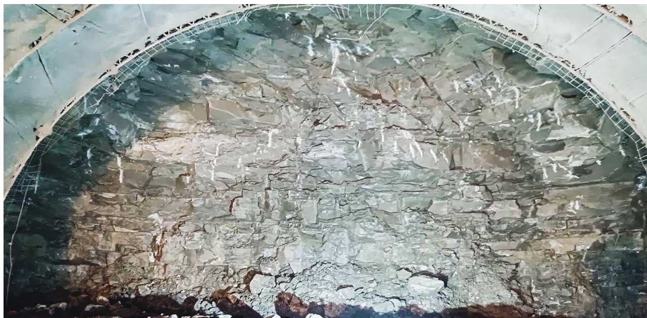
Fig. 2: Siltstones at the headwall of the Homole tunnel
