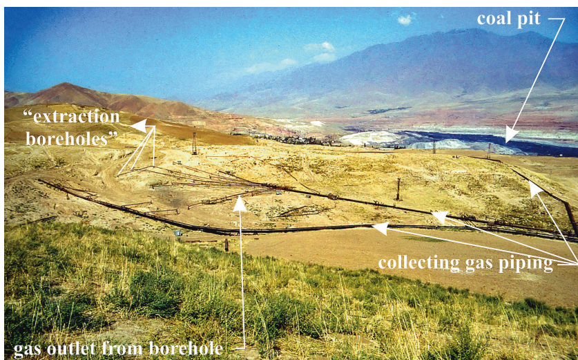
Fig. 5: View of “extraction boreholes” and gas piping
