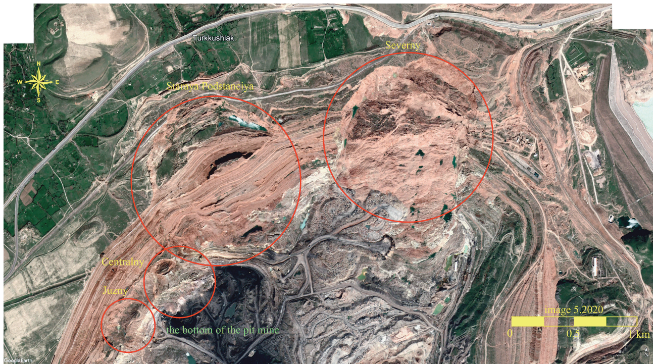
Fig. 10: Slope failures on the north and northwest walls of the pit
