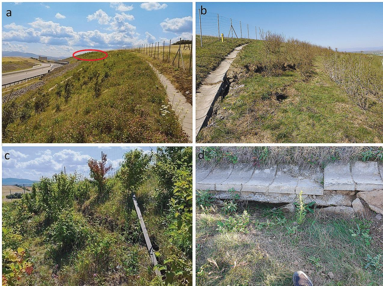
Fig 2.: a) The cut of the R4 expressway with a marked zone of a landslide, b) landslide above R4, c) a shear zone, d) destroyed dewatering surface element.
