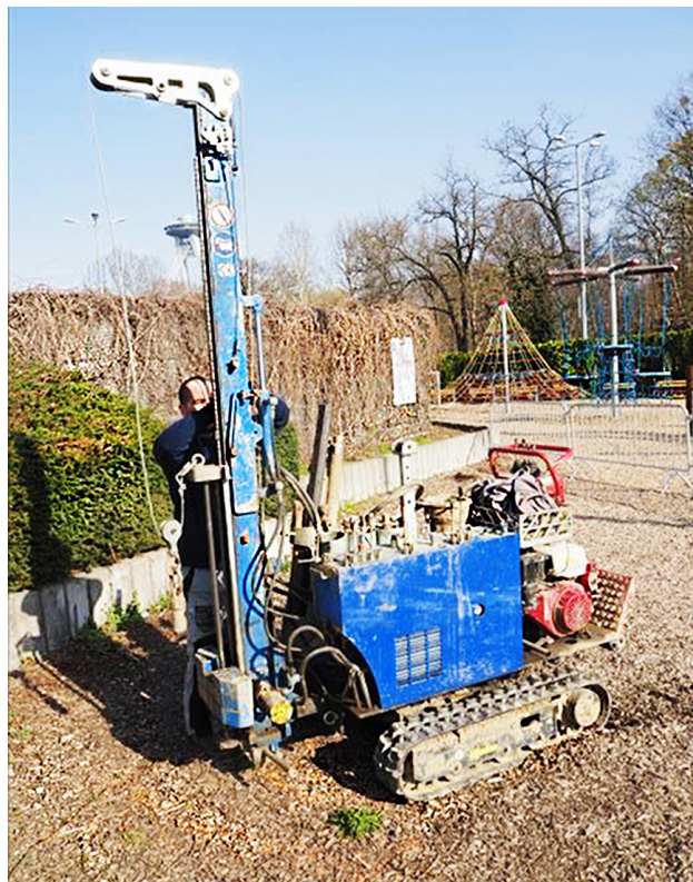
Fig. 4. Drilling of monitoring wells
