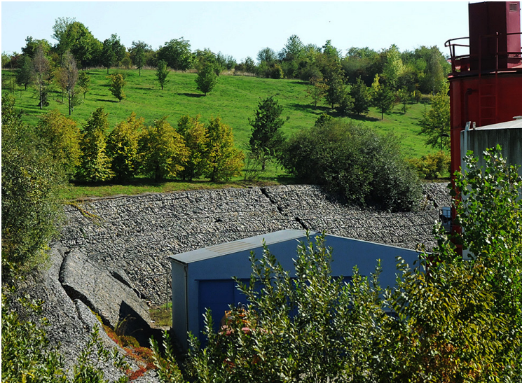
Fig. 10. Pohnava, Cimburkova Street, landslide behind Tesco department store after its stabilization in 2004.
