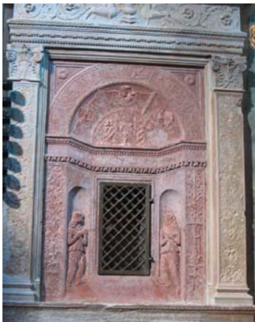
Fig. 1. Early Renaissance tabernacle in the upper church of the St. Emmeram's Cathedral. Pilasters, top and bottom ledges were carved from yellowish crinoidal limestone, the inside part from red nodular limestone, both from northern Hungary.
